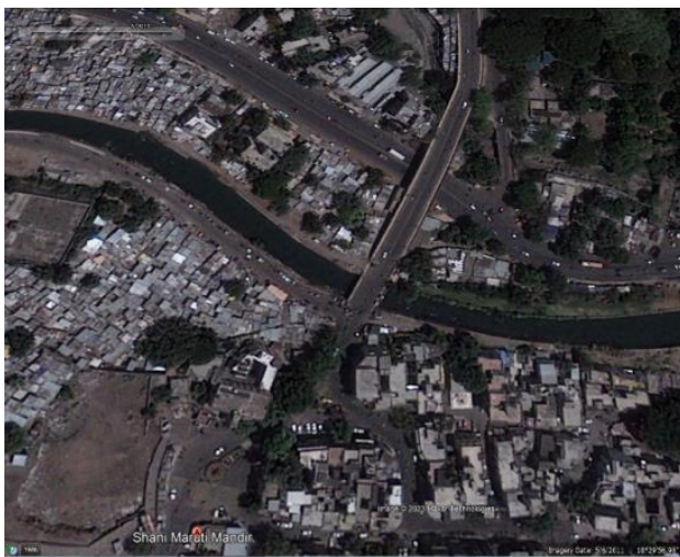
Timeline: 2011 (canal reaches its halfway point in term of construction)
