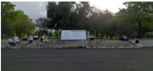
Absence of Ramp and Grab Rail
