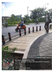
Tactile paves and kerb ramp
